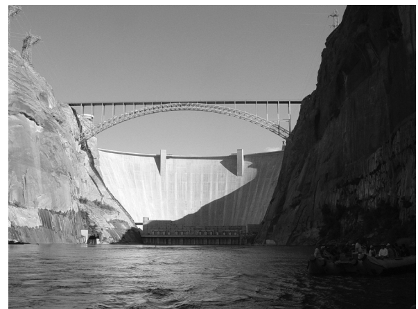
Glen Canyon Dam
